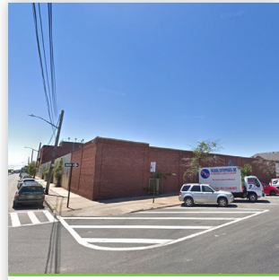
1340 EAST BAY AVE
